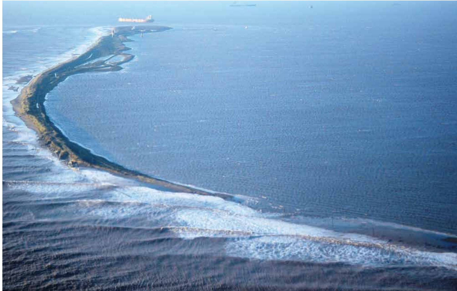
The storm surge breaches the narrows on the peninsula © Environment Agency copyright 2013. All rights reserved
